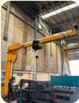
Jib Crane after
