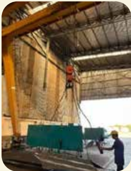
Jib Crane before
