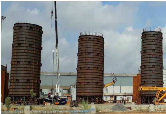
Site Installation underway
