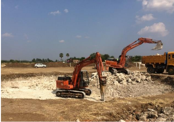
Site Installation underway
