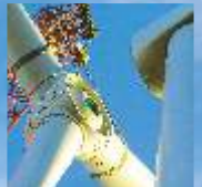
ERECTION OF WTG
