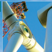
ERECTION OF WTG
