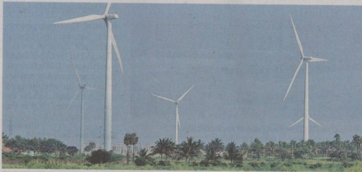
TIME FOR OVERHAUL: As per the Ministry of New and Renewable Energy report, most of the wind turbines installed till the year 2000 are below 500 kW capacity. — FILE PHOTO
