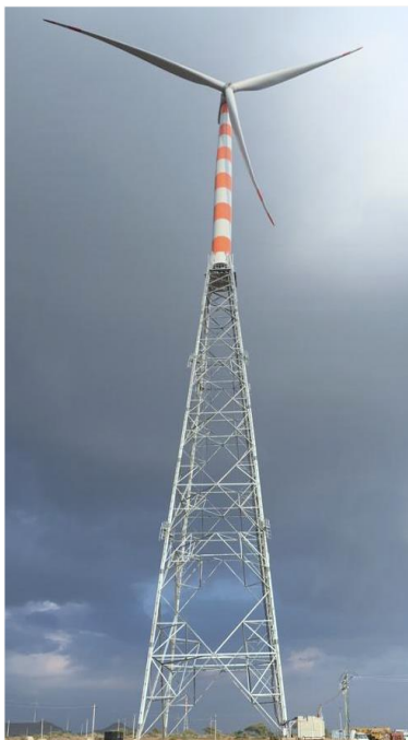
S120 – 140 HLT (Dec '18) Hybrid Lattice Tower
