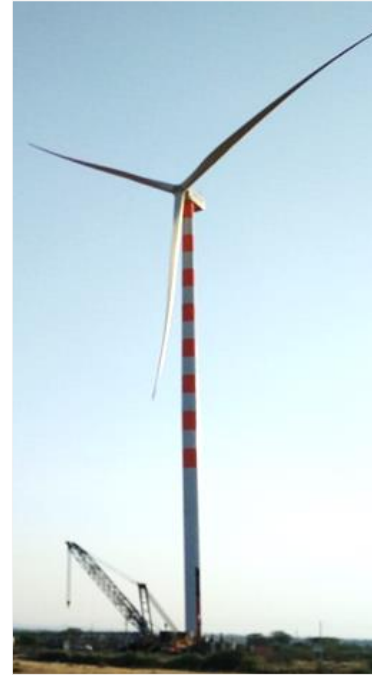
S120 – 120 STT (Jan '19) Smart Tubular Tower
