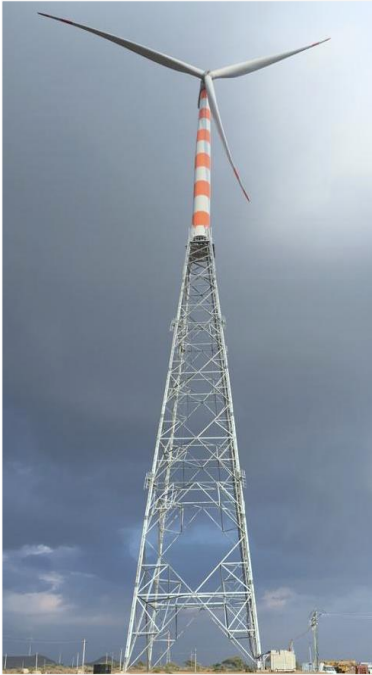
S120 – 140 HLT (Dec '18) Hybrid Lattice Tower
