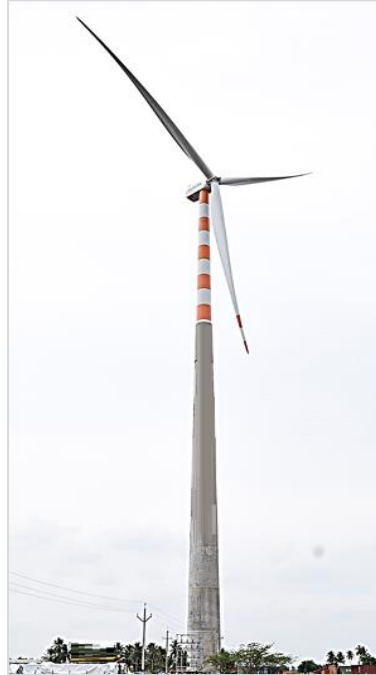
S120 – 140 HCT (Sep '18) Hybrid Concrete Tower
