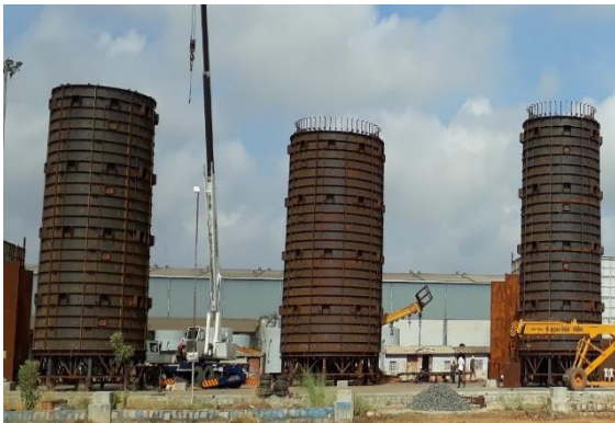
Site Installation underway
